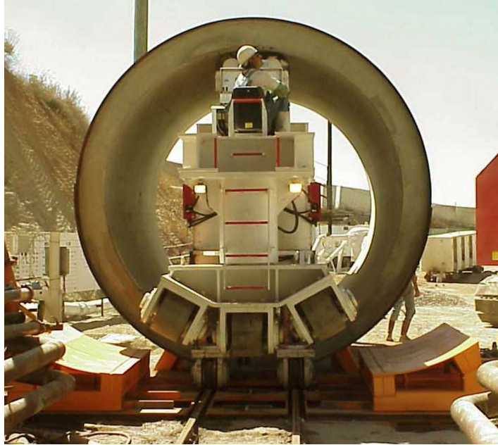
Figure 1. 144-in. Diameter Composite Wall Tunnel Liner
