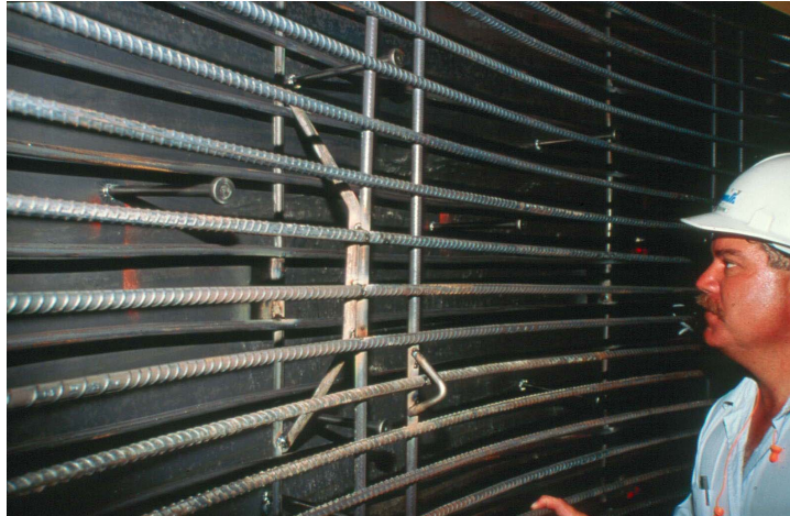
Figure 3. Reinforcing Cages and the Nelson Studs inside the Cylinder
